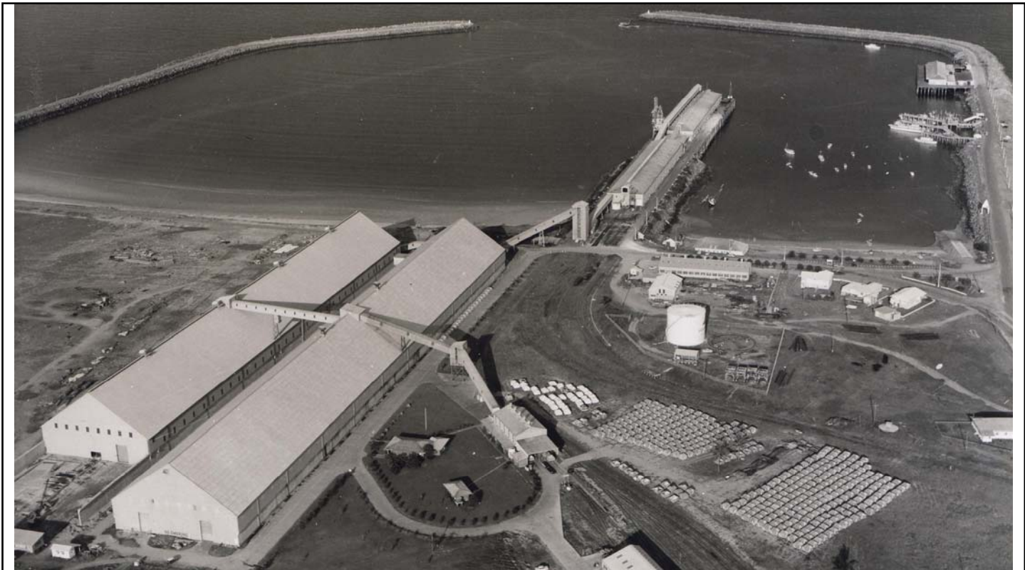
Mackay Bulk Sugar Terminal (RHSQ collection)
