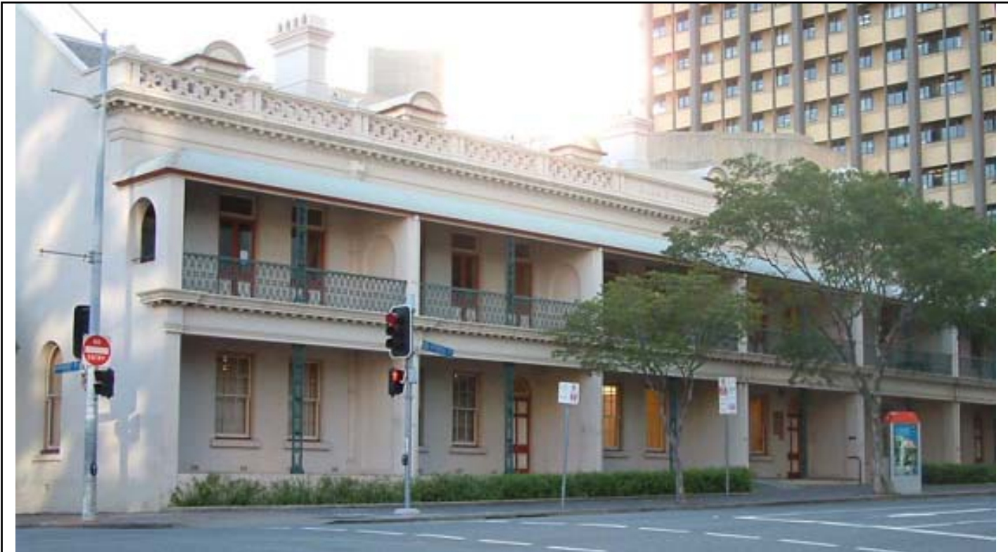
Harris Terrace, George Street Brisbane first occupied in 1867; above photograph by Allan Bell, September 2007
