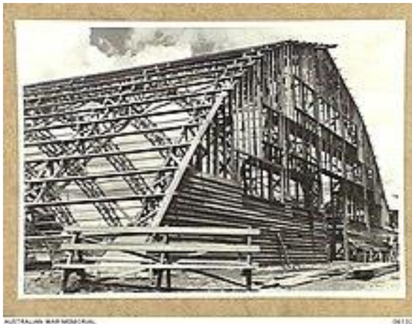
Australian Army canteen "igloo" under construction in Atherton, Queensland, 1943
