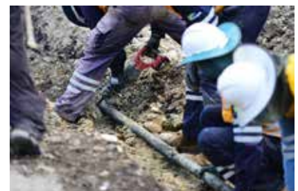
Workers removing Edison lighting tubes from William St, February 2018 (ABC News)
